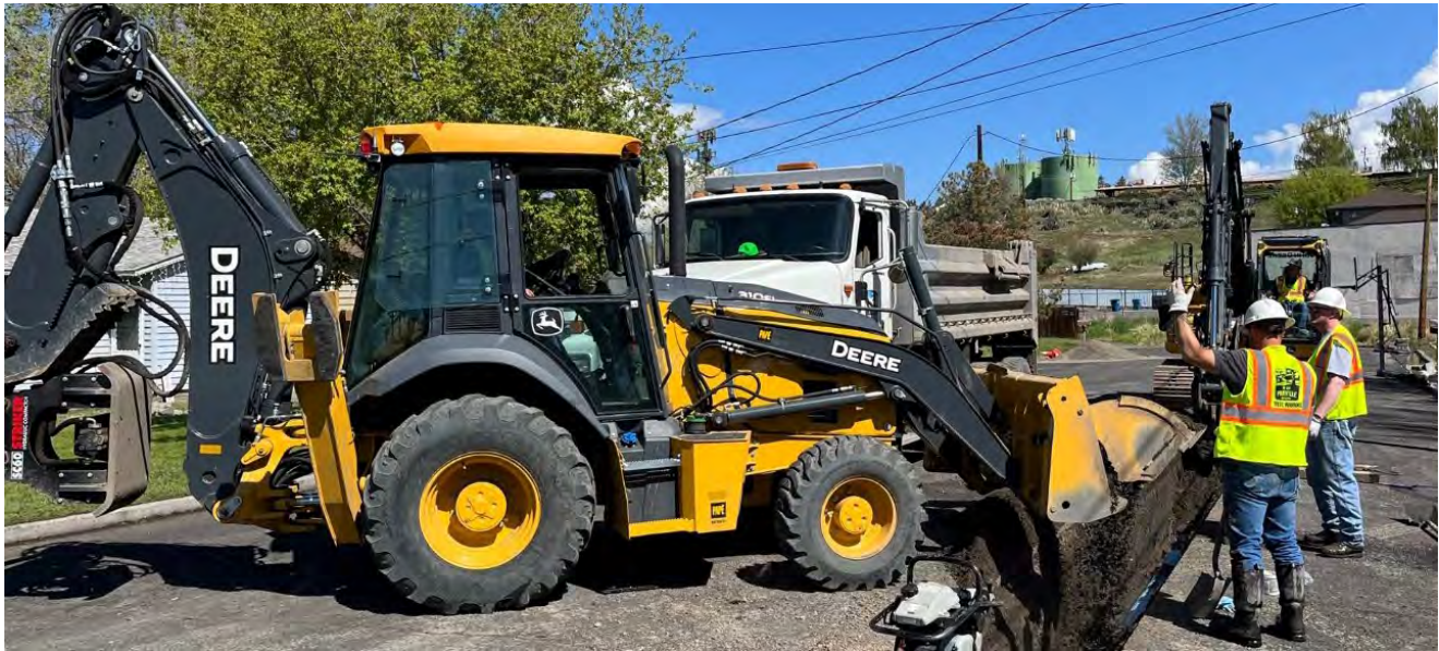
The Dunham waterline project in August 2023
