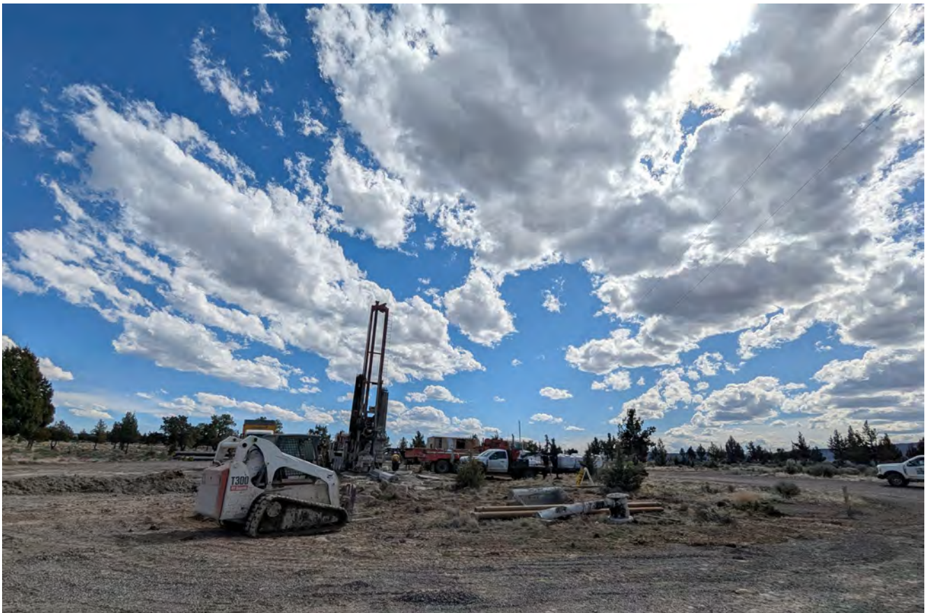
Well drilling in March 2025
