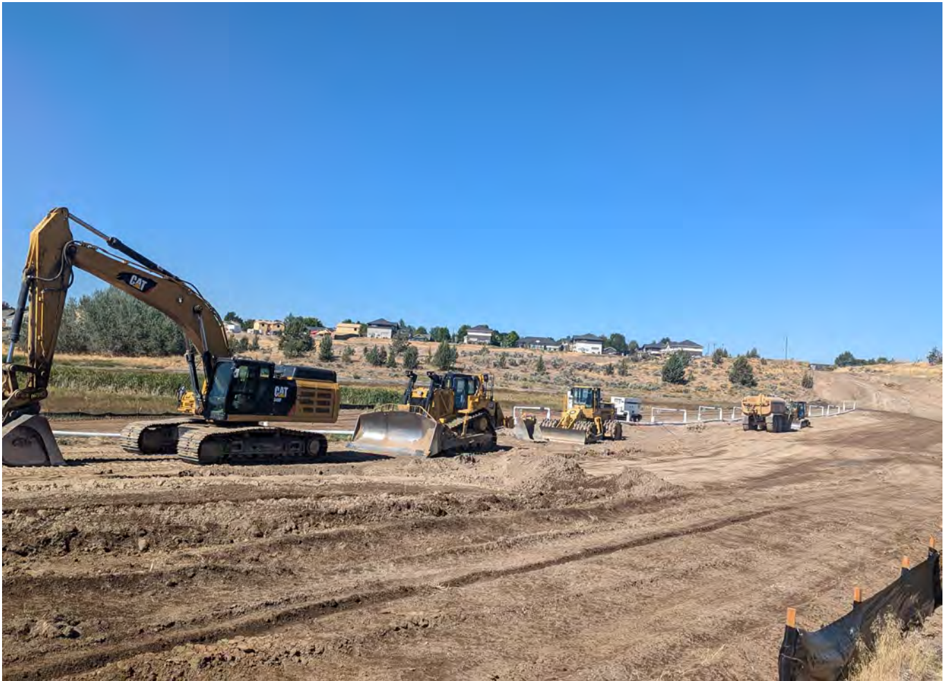
Combs flat extension project in August 2024
