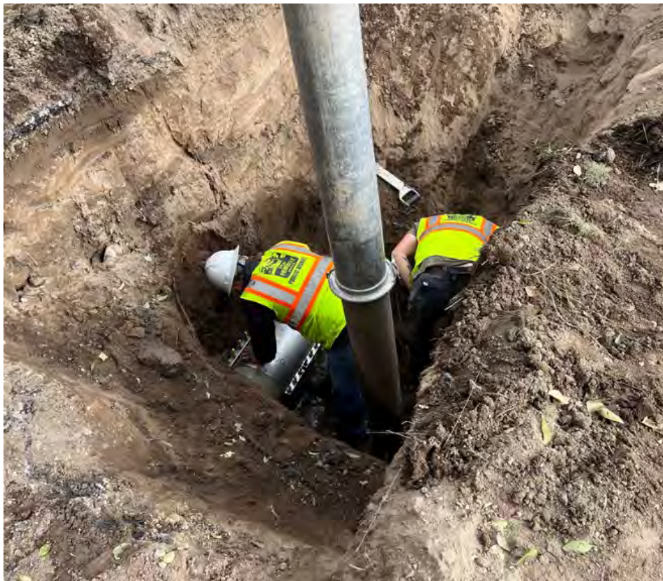
Utility Line work being done in BN 25
