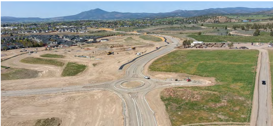
The Combs Flat Extension project in April 2025.
