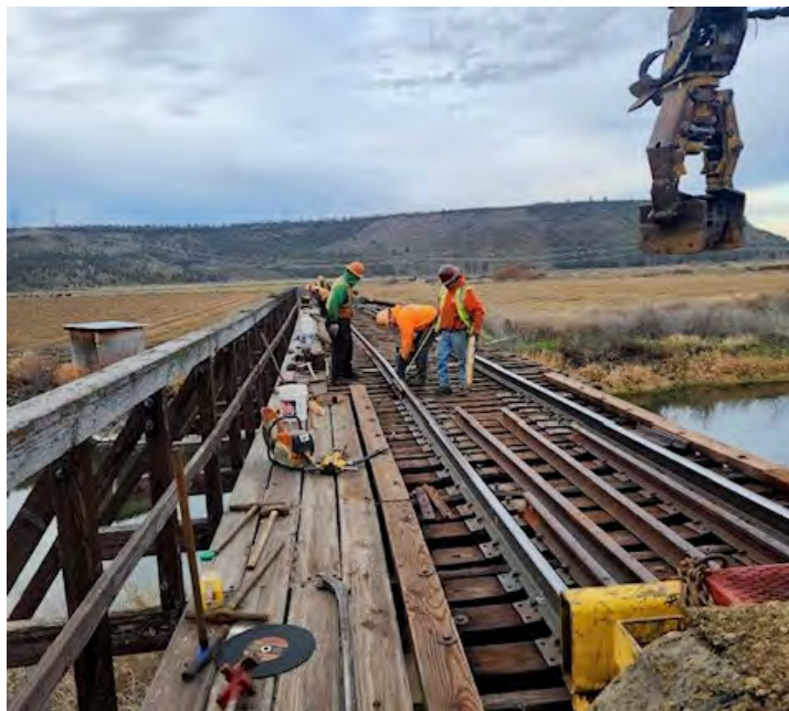
Railroad Bridge work being done in December 2023
