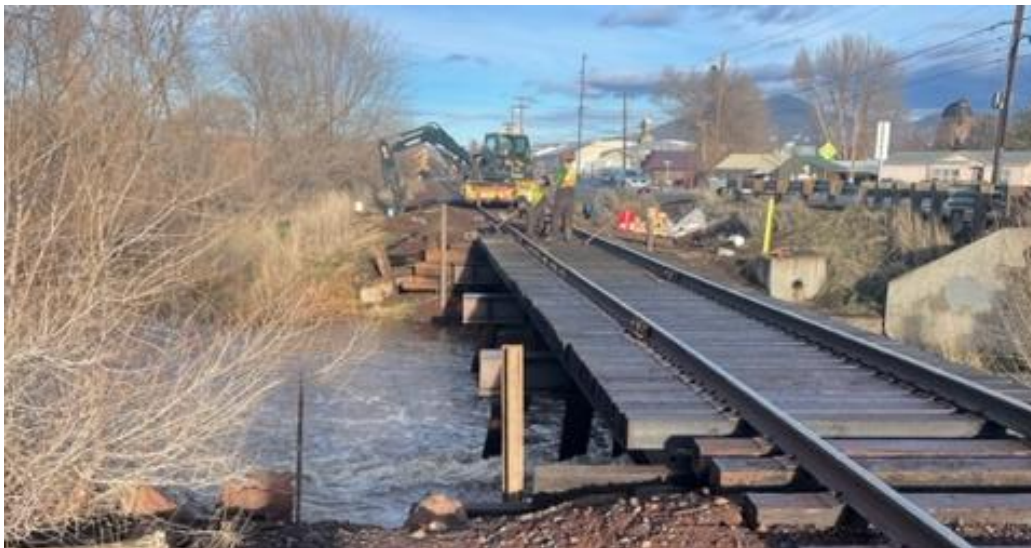
Bridge work being done during the third quarter.
