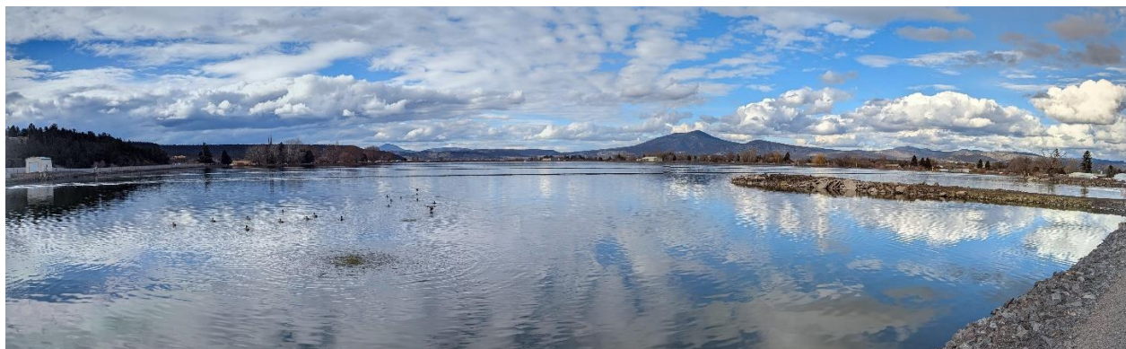
Wastewater treatment facility in February 2024
