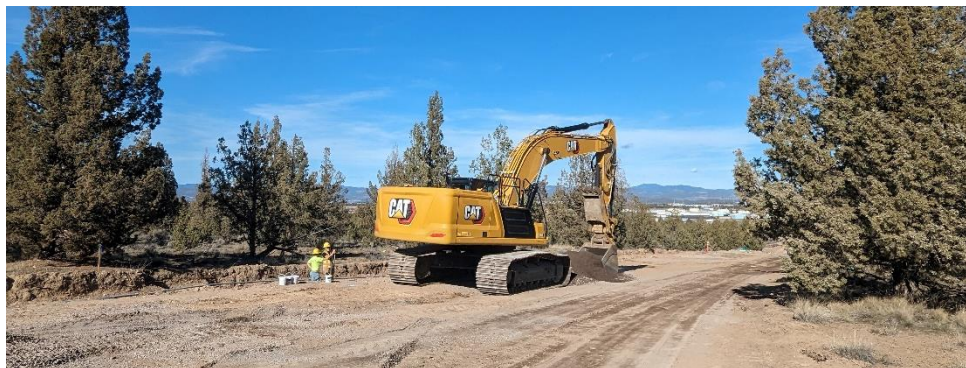
Waterline extension project work during the third quarter.
