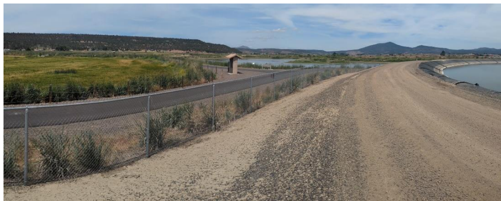
Wastewater treatment facility in June 2024
